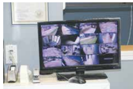
Security cameras cover the facility.
