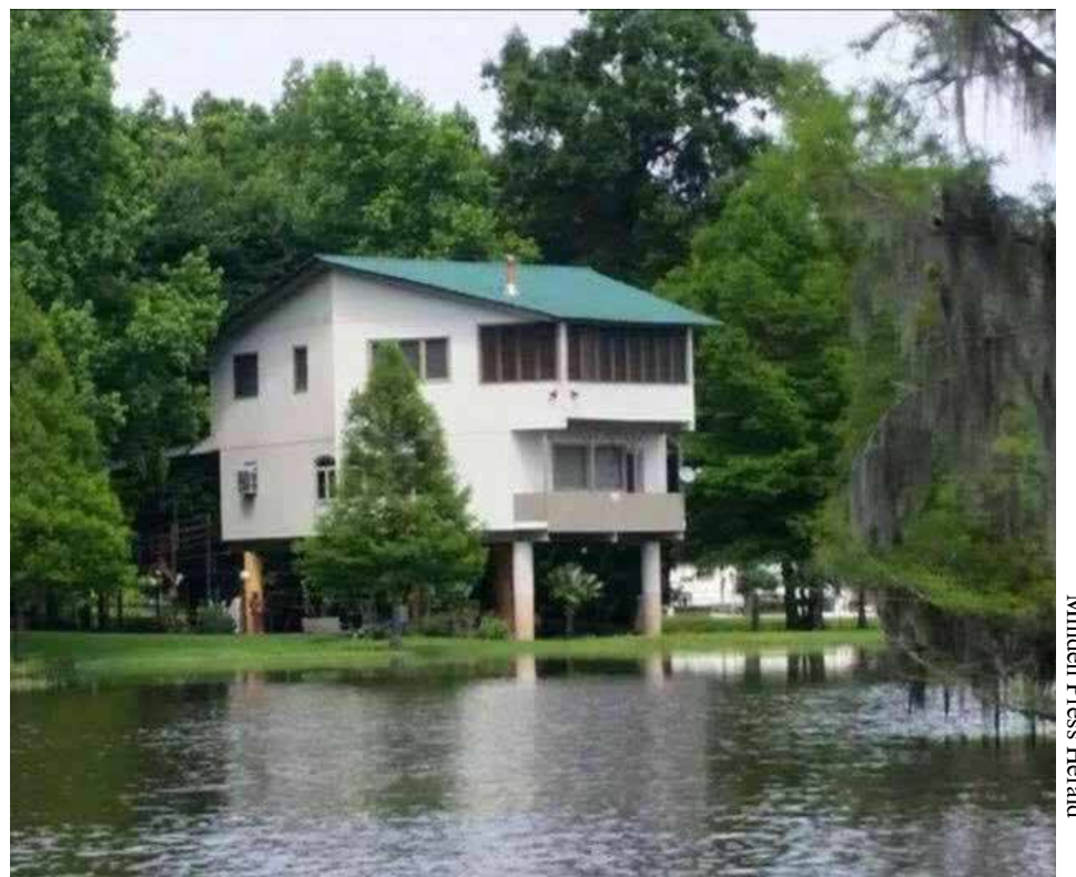
Catherine Hunt’s house at Lake Bistineau. Houses like this now have protection.
