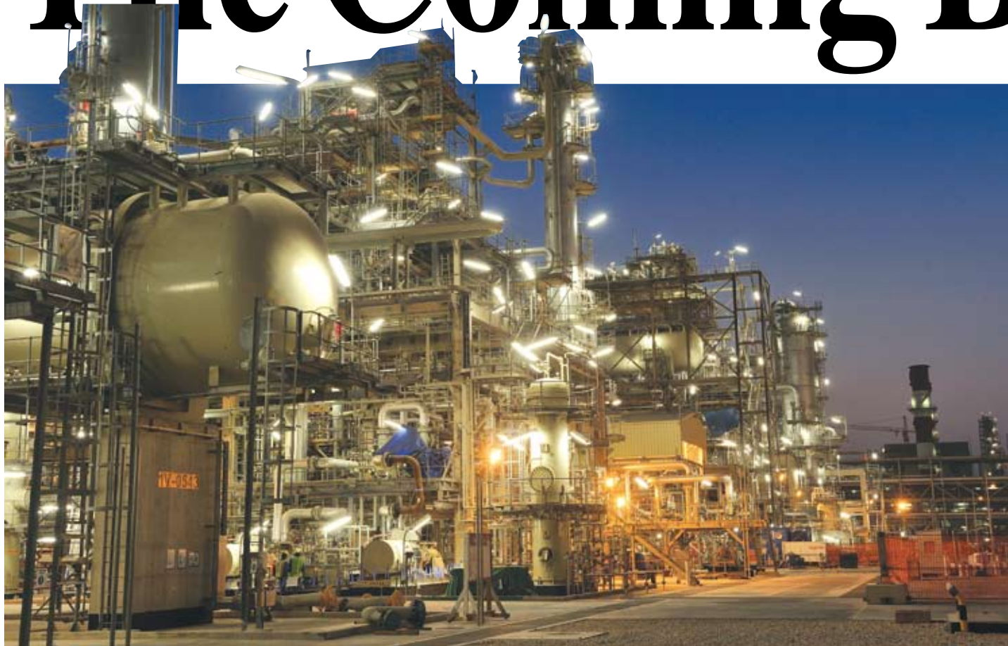
SHELL GAS-TO-LIQUIDS PLANT IN QATAR — Revolutionary technology, which converts natural gas to synthetic gasoline and can be used in automobiles without any special devices, is used in this Shell plant in Qatar and may be coming to South Louisiana.
