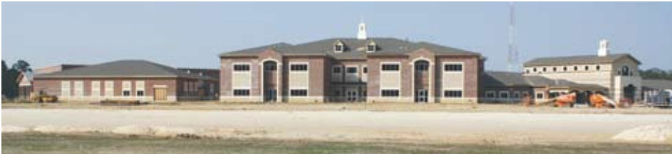
For the new Central School Complex, it's moving-in time.
