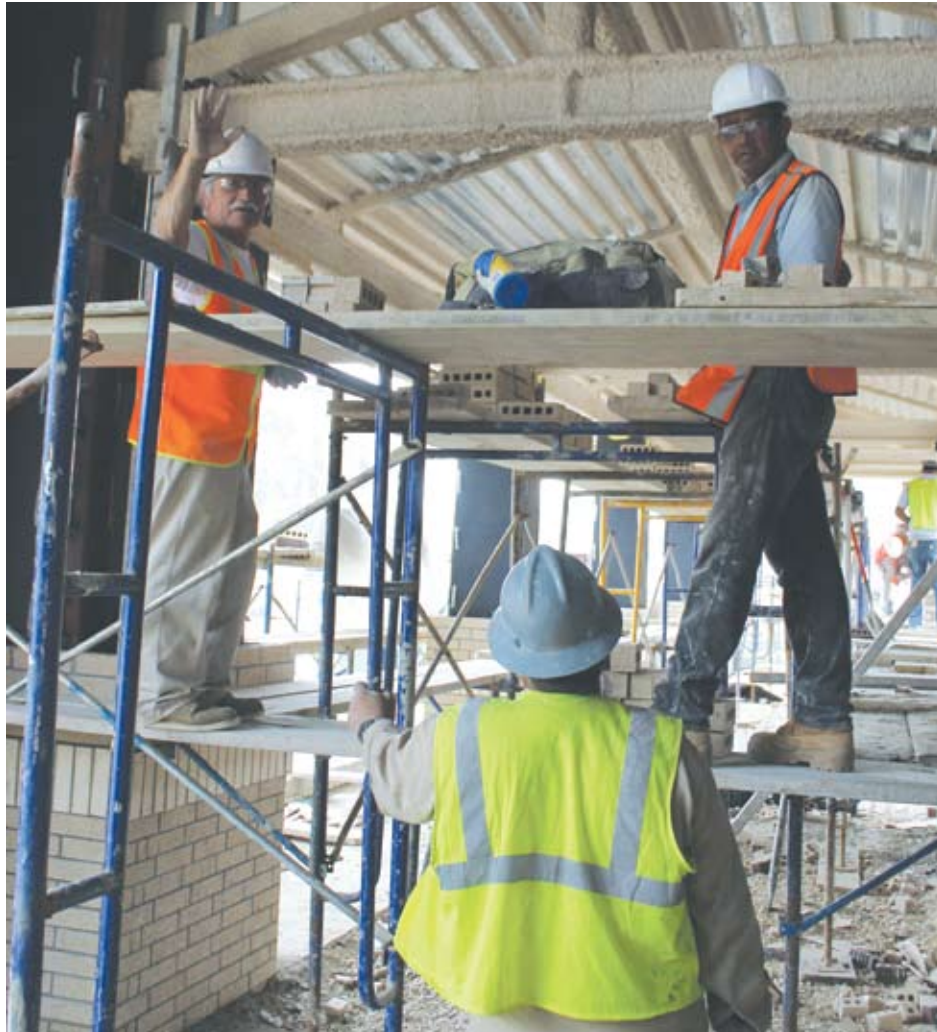
Men working on the new School Complex
